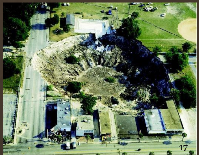
This image shows a sinkhole, formed as a result of the karst system underground.
